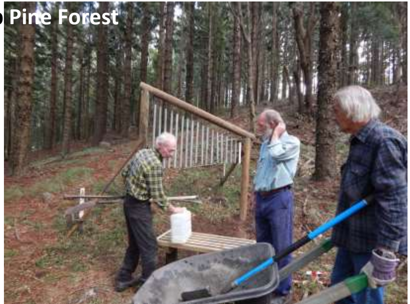
Will, Don and Graham installing the chimes
